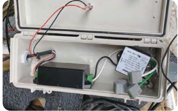
1. Run AC cable and conduit to the box according to NEC Article 300 and any applicable local codes. The gland accepts 1/2" conduit.
