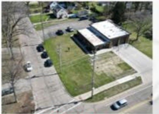
STATION 6 NEW ADDITION & RENOVATION
