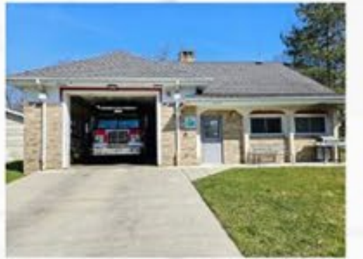
STATION 5 NEW ADDITION & RENOVATION
