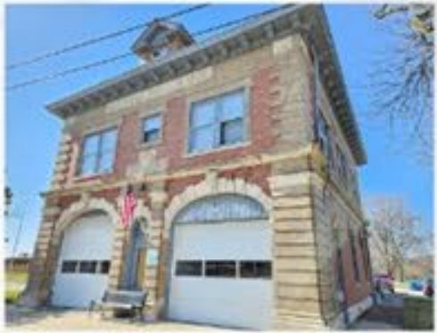
STATION 2 NEW STATION
