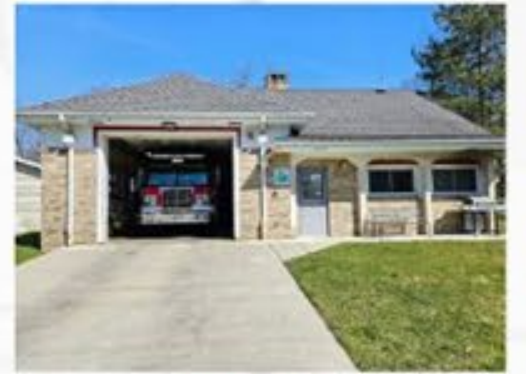
STATION 5 NEW ADDITION & RENOVATION
