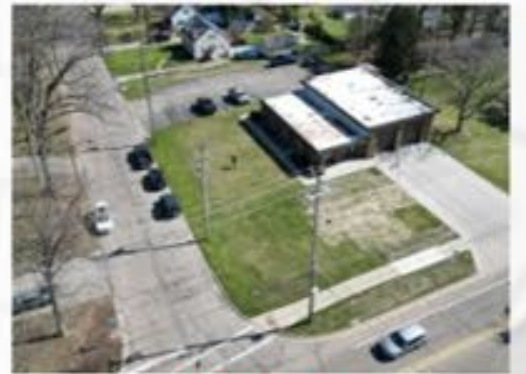
STATION 6 NEW ADDITION & RENOVATION
